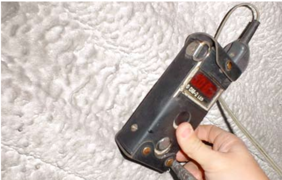
ILLUSTRATION 9: ULTRASONIC TESTING OF THE STEEL VERIFIED THAT NO MEASURABLE SECTION LOSS HAS OCCURRED.
