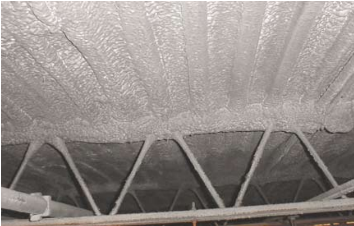
ILLUSTRATION 3: VIEW OF TEST REGION SELECTED, LOCATED IN PROXIMITY TO HYDROCHLORIC ACID PROCESS.
