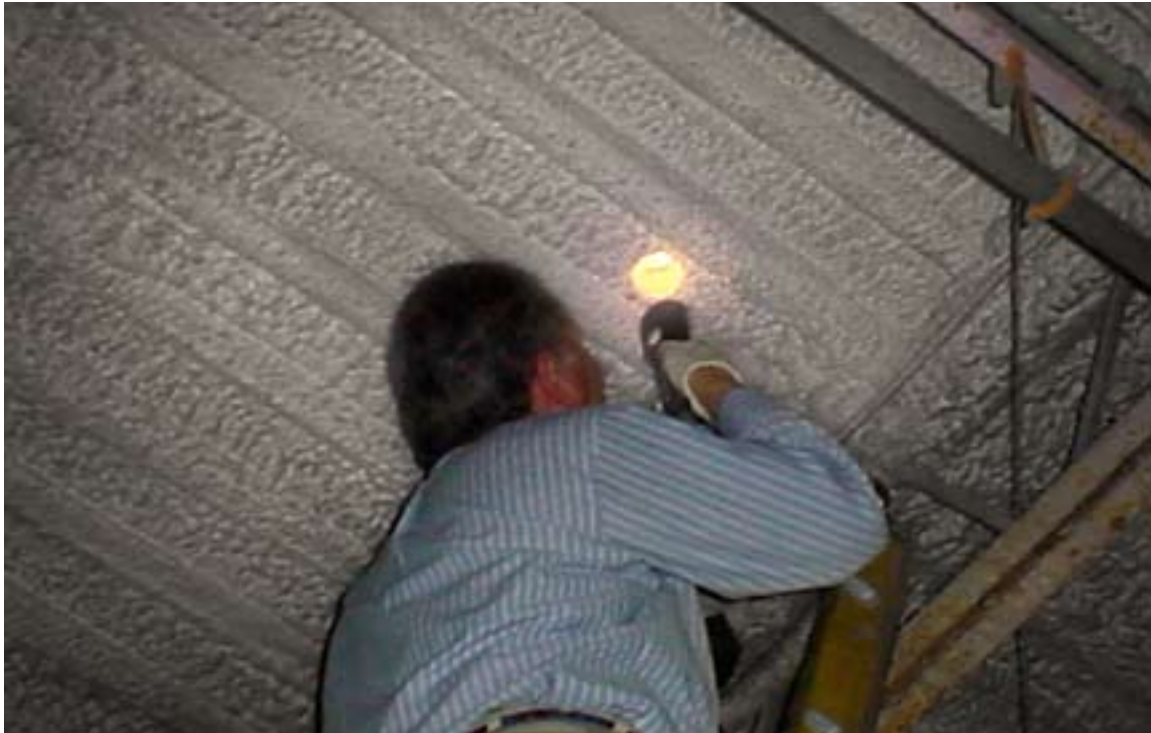
ILLUSTRATION 5: VIEW OF SUBSURFACE SUBSTRATE CONDITION SURVEY.
